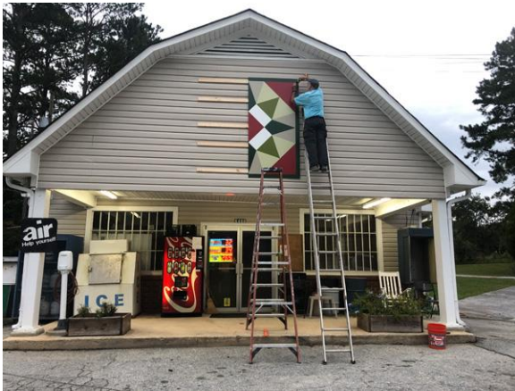
Figure 9 – Install wood strips to support the barn quilt on uneven surfaces
