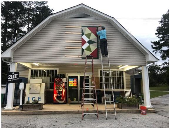
*Figure 9 – Install wood strips to support the barn quilt on uneven surfaces*
